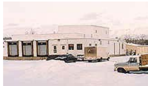
Turnkey plant in Mt. McKinley, Alaska
