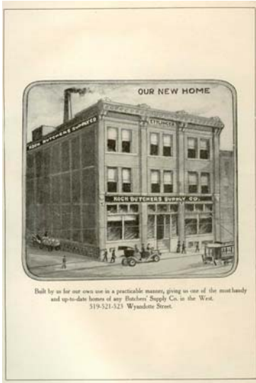
New building erected at Fifth and Wyandotte in 1916
